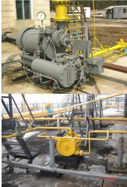
Expansion turbine - an electric power generation unit as a part of jet-reactive (ET-JRT) and vortex (ET-VT) turbines is used to produce electric power out of compressed gas or steam due to numerous power leaks in places where regulators and pressure reducers are mounted.
